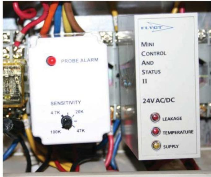
*Flygt Retrofit Relay installed in a Flygt panel next to the MiniCAS permits use of SH Pump with their Panel.*
